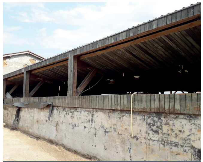
Photo 20 - Installation de volets
